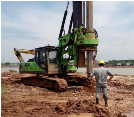
Hydraulic Rotary Piling
