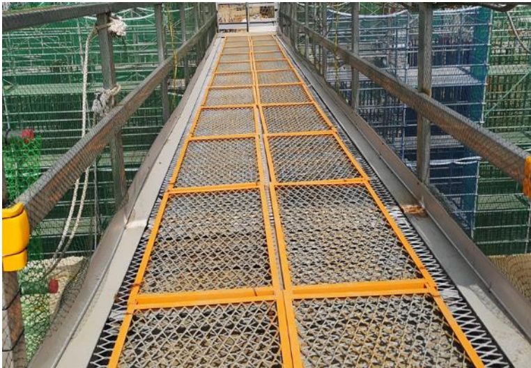
Drainage system mockup to prevent environmental pollution into public drainage system and designated safe walkway
