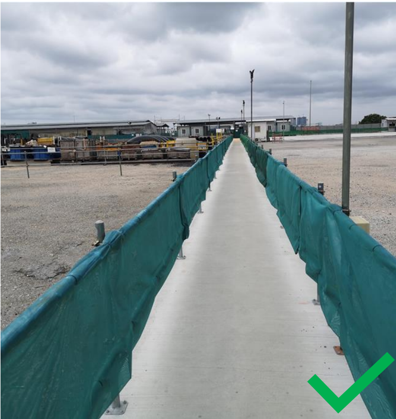
Best Practice: Provide designated paved clean walkway with guardrail.
