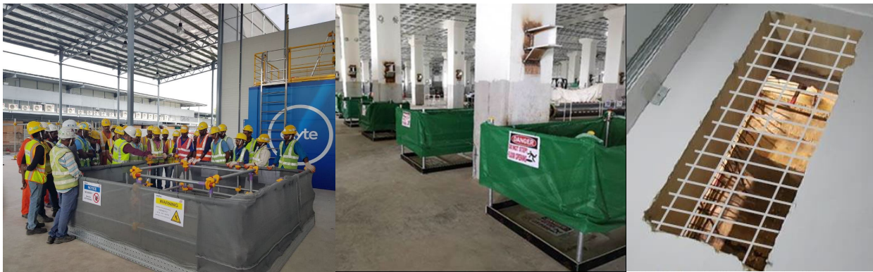
Figure 3 Floor Opening Floor Opening mockup with guardrails, opening cover, toe board and warning signages for awareness training
